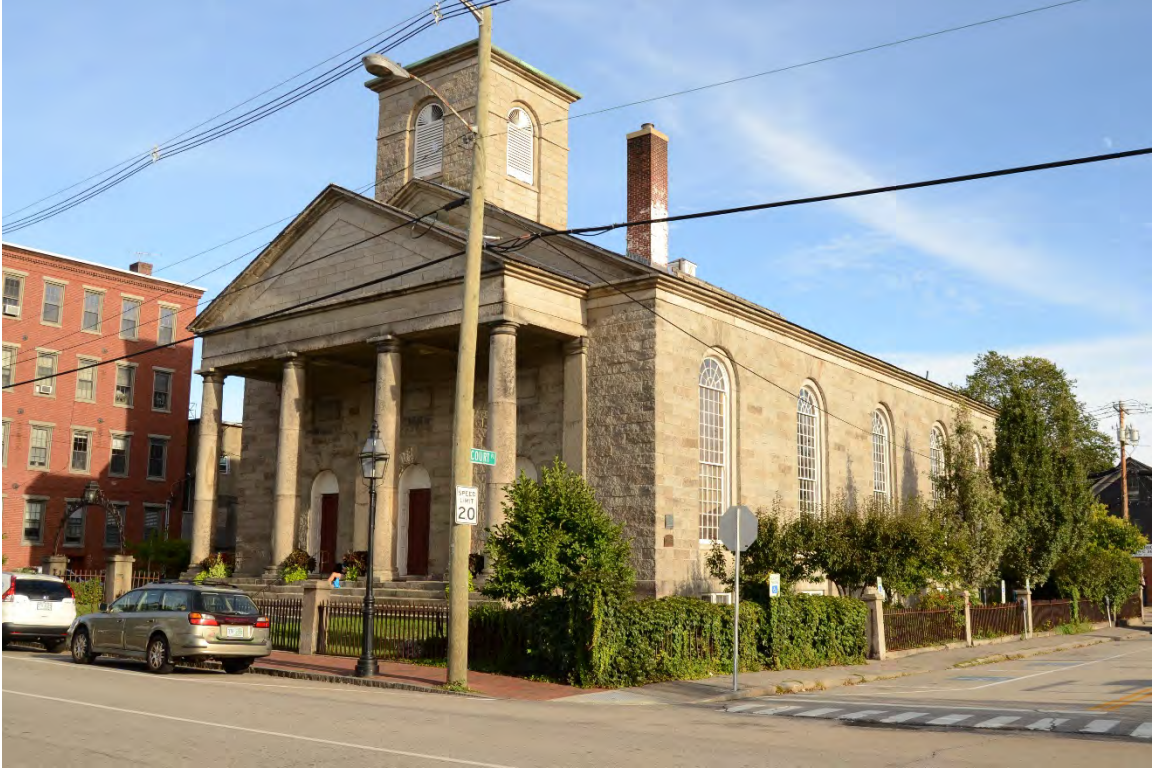
Photo 38. South Parish, 292 State Street (NR listed), looking southeast.
