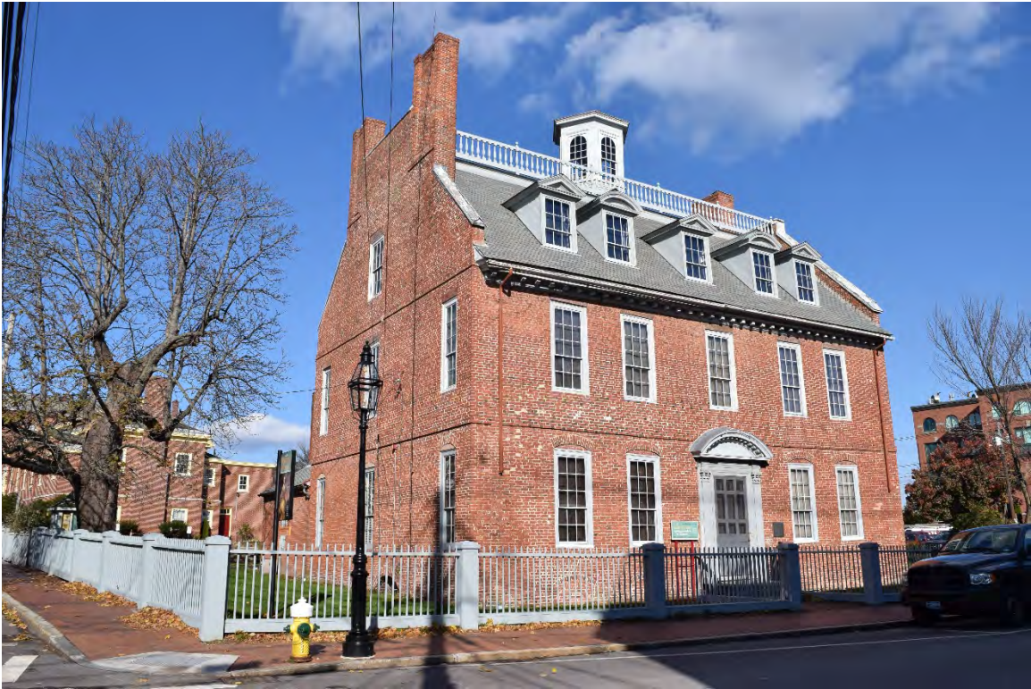
Photo 7. The MacPheadris-Warner House, 150 Daniel Street (NHL listed), looking north.
