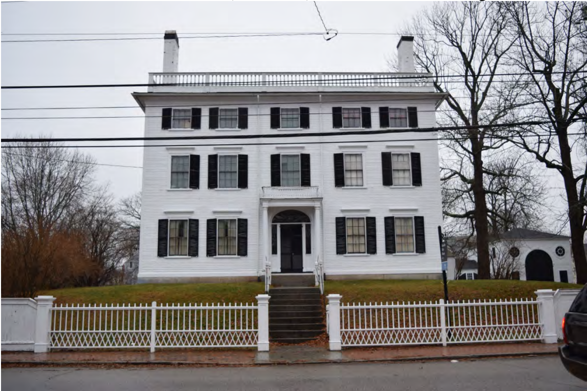
Photo 23. Rundlet-May House, 364 Middle Street (NR listed), looking northwest.
