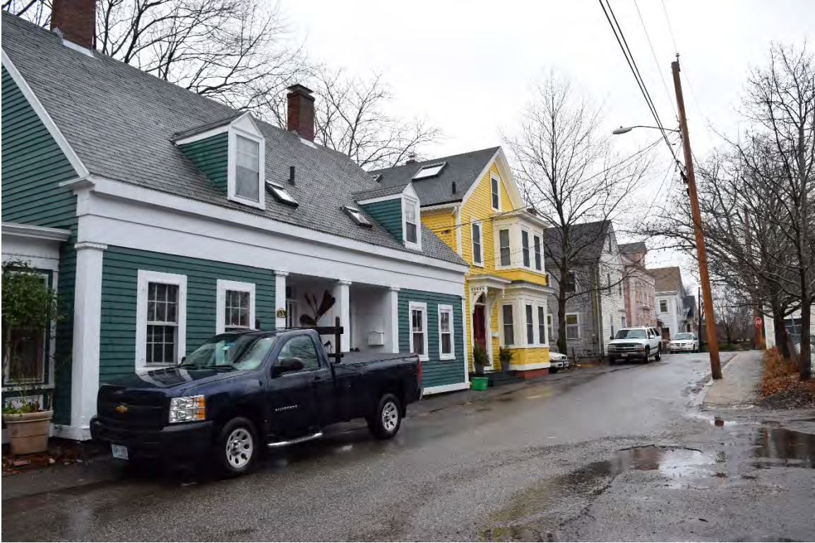
Photo 42. Winter Street, looking northwest from the intersection with Chatham Street, showing (l-r) 22-24, 30, 40, and 48 Winter Street.
