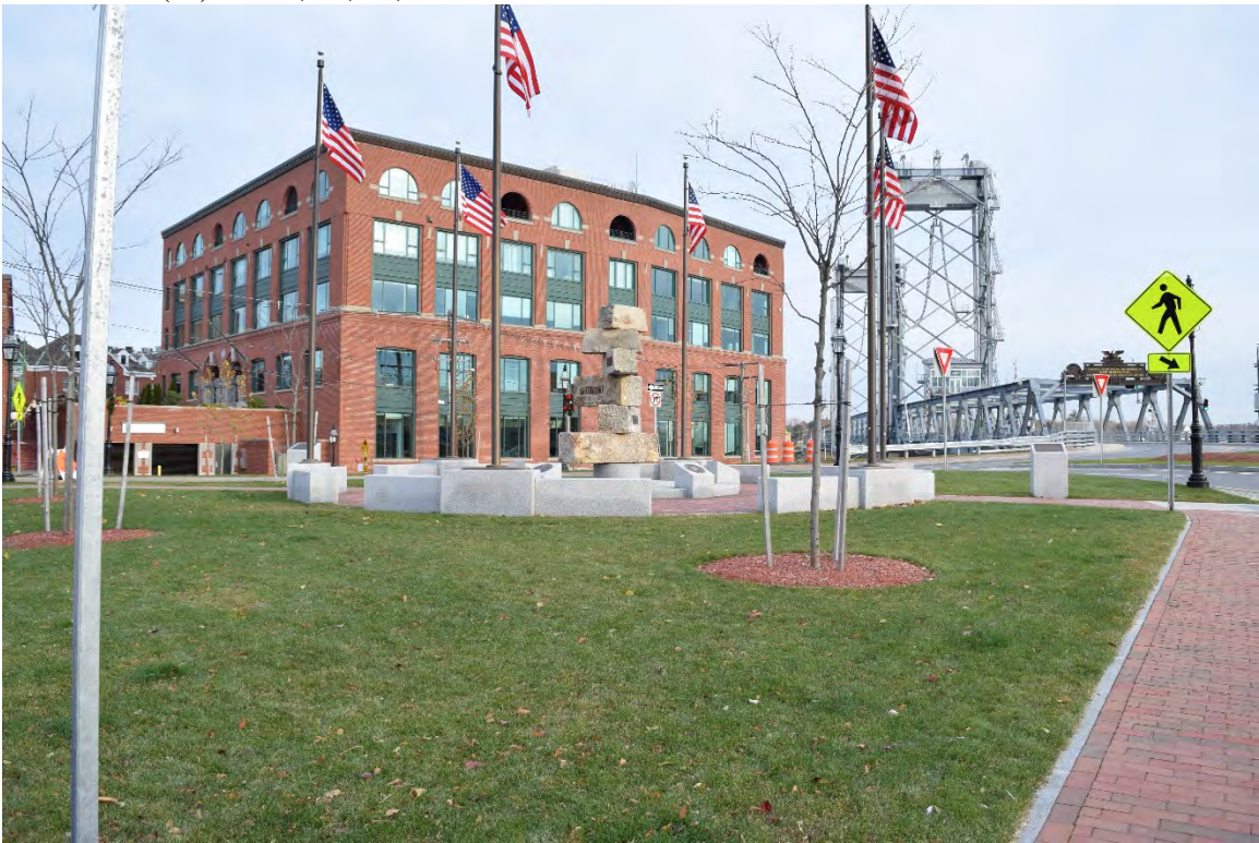
Photo 43. Portsmouth Memorial Park on Wright Avenue and the former Portsmouth Gas and Electric Light Company Power Station, 1 Harbour Place, with Memorial Bridge (outside district) in background, looking north.
