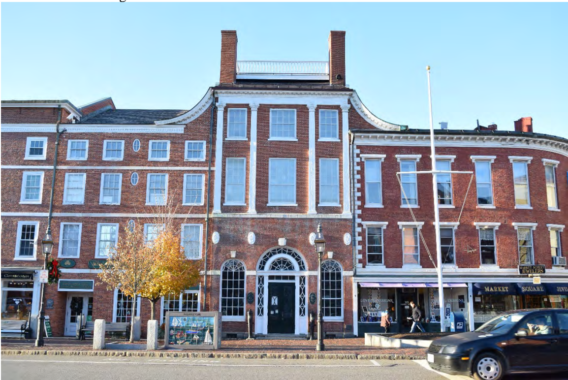
Photo 19. Portsmouth Athenaeum, 9 Market Square (NR listed) and surrounding buildings on Market Square, looking northwest.
