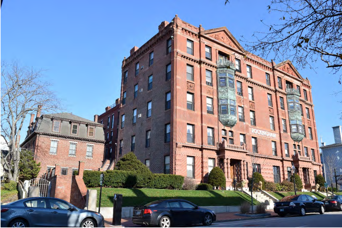
Photo 39. The Rockingham Hotel, 401 State Street (NR listed), looking north.
