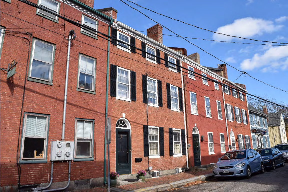
Photo 36. Rowhouses, 7-9 Sheafe Street, looking northeast near the intersection with Penhallow Street.
