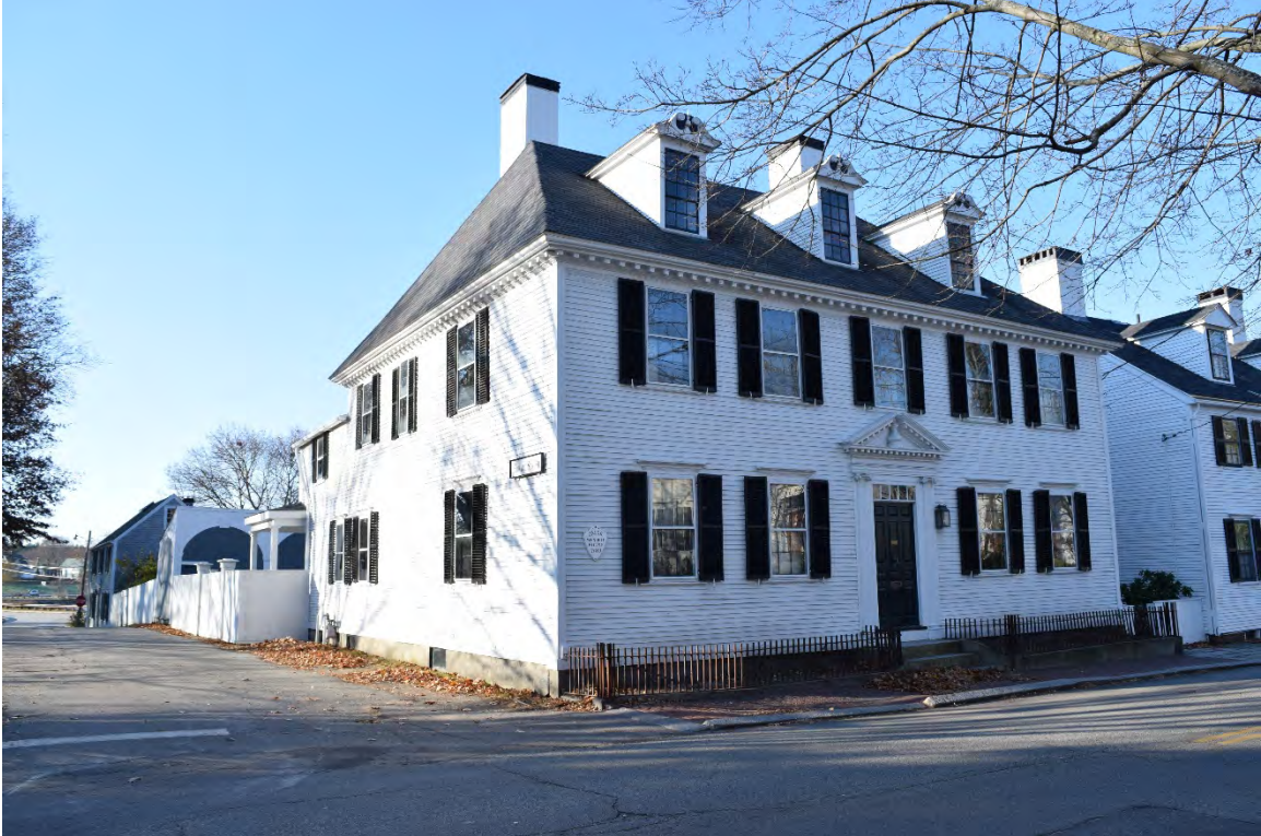
Photo 29. Jacob Wendell House, 222 Pleasant St, with a Chinese Puzzle Garden behind the house looking southwest.
