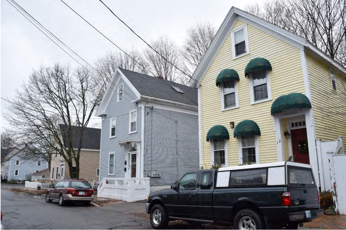
Photo 40. Union Street, looking southwest from near the intersection with Islington Street, showing (r-l) 12, 20, and 32 Union Street.
