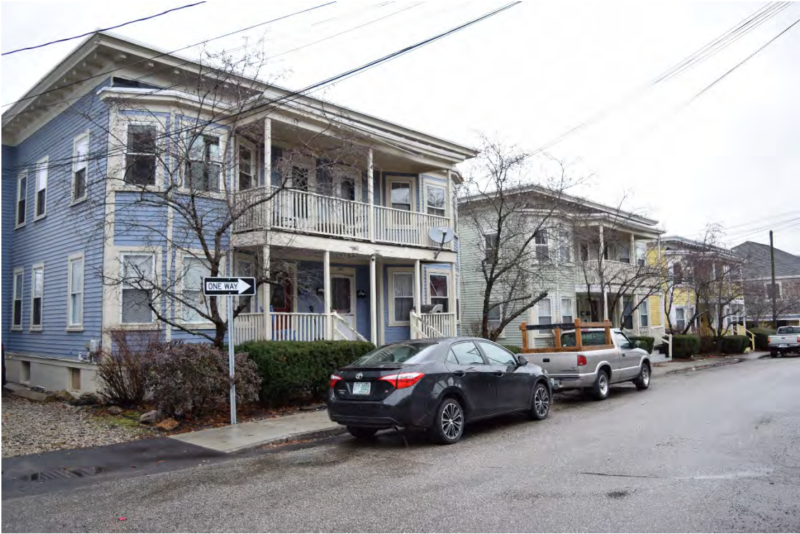
Photo 8. Hanover Street, looking northeast from the intersection with Pearl Street; 349–351 Hanover Street is in the foreground.
